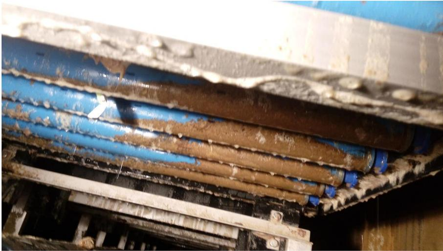
**Figure 2.** Sludge intrusion into diffuser
